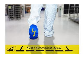
Generation 3 coating consists of an electrically conductive primer and EpiMax 333WB-EC as a high gloss coating with electrostatic discharge properties.
