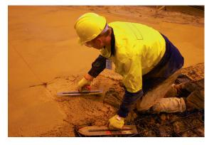
Sub-floors can be topped with performance epoxy or polyurethane cement floor protection systems. Typically these floors are installed in food production and packaging areas, commercial kitchens, manufacturing and engineering and workshops.
