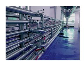
Floors in food premises must be able to be cleaned effectively and thoroughly, must not absorb grease, food substances or water, harbour pests, and should be installed so as not to cause pooling of water.
