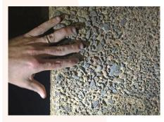
The spray application of EpiMax 655 will address these conditions and provide a sound, relatively flat surface for further coating application without promoting pinholes due to air expansion from within the concrete.
