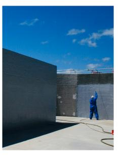
Irregular surfaces can lead to protective coating discontinuities via the formation of pinholes and voids. Additionally, they will not allow protective coating film thicknesses to be measured accurately.
